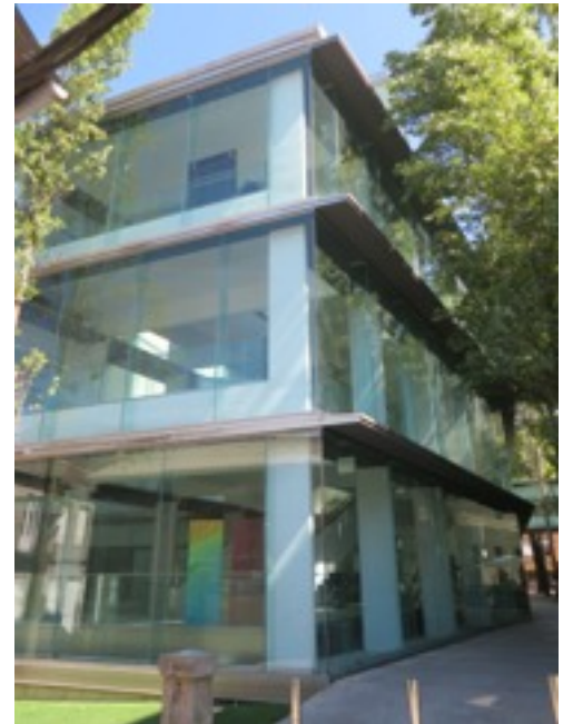
The main building of the Pontevedra Museum
